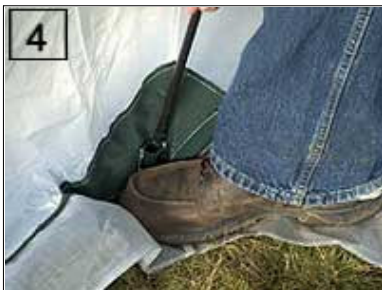
Step 4: Begin assembling the fiberpoles by inserting one capped end into the pocket near the floor. Insert the other end into the pocket directly across from the first.
